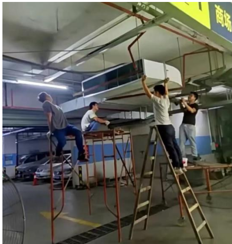
Figure1 workers are installing the ventilation system in underground garage
